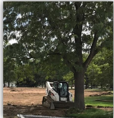
**Figure 3.** Heavy equipment traffic compacts soils.
