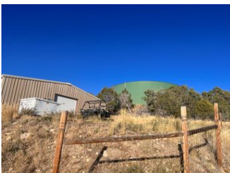
Existing Lamborn Finished Water Tank
